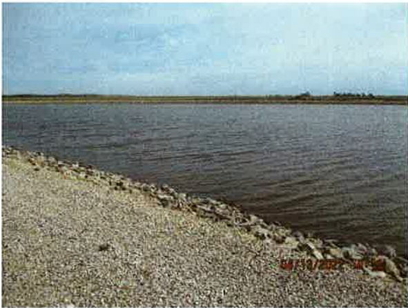
Photo Taken: 4/13/2022 10:13:33 AM Secondary Cell 2, Looking northeast
